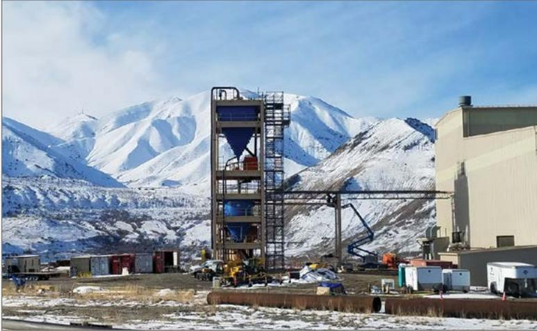
**Eriez HydroFloat uses a novel aeration system to disperse fine bubbles into a fluidized-bed environment.**
